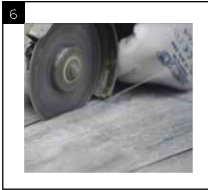
6. Grinder equipped with diamond disk
