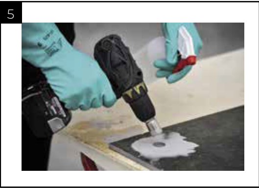
5. Diamond tool for wet drilling
